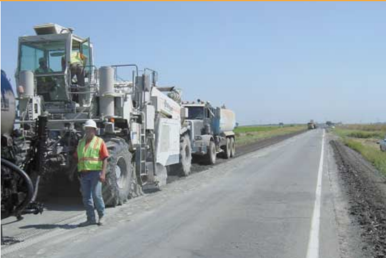
Two WR 2500s foam-stabilize base in echelon in Colusa County, California
