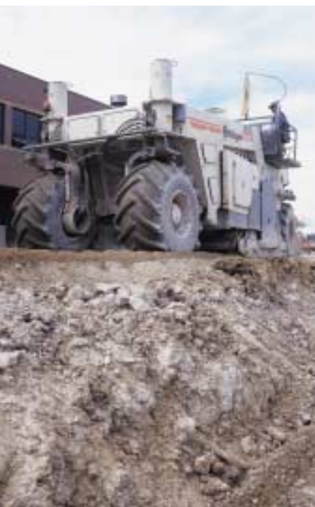
Lime-stabilizing in Broomfield, Colorado
