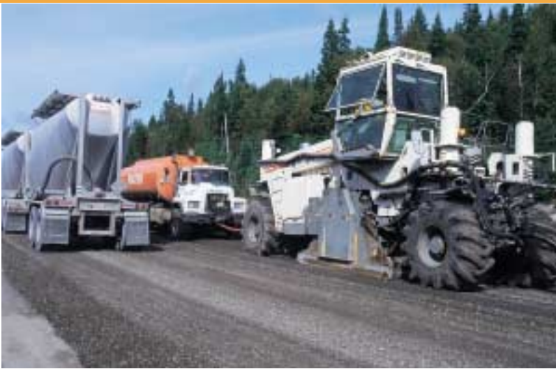
Newly stabilized base stands up to cement truck immediately
