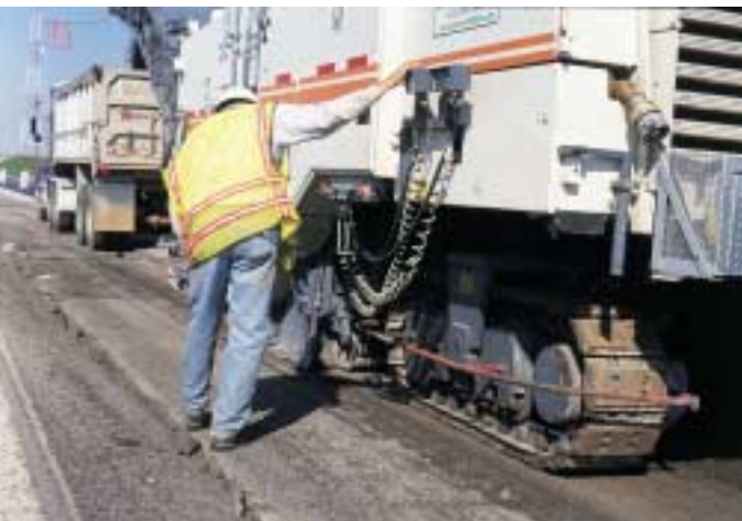
Payne & Dolan crew checks depth of cut
