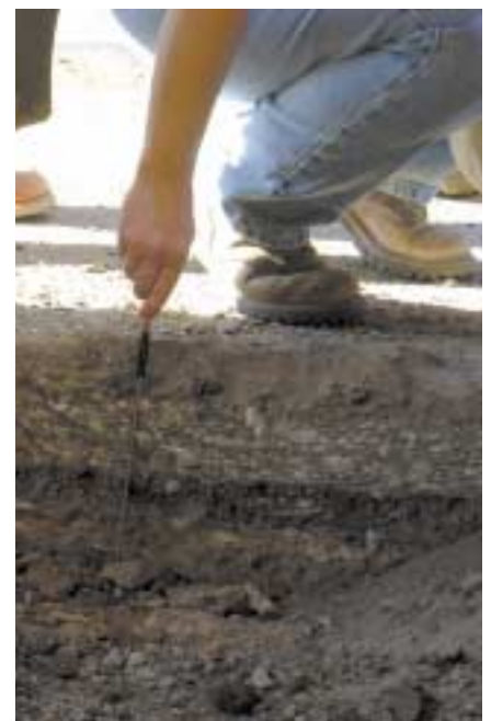
Existing pavement recycled to depth of 9 inches
