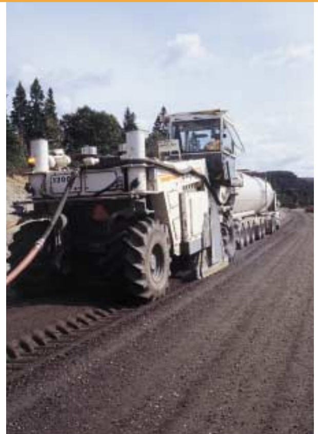
WR 2500 at work in provincial park
