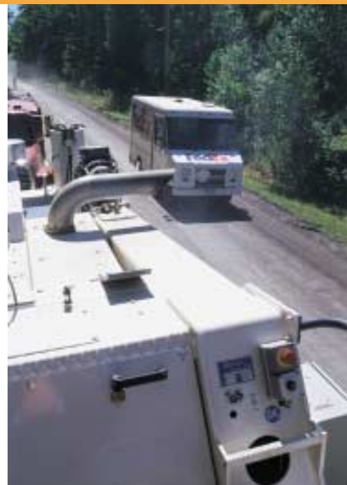
Courier truck delivers using freshly foam-stabilized road base
