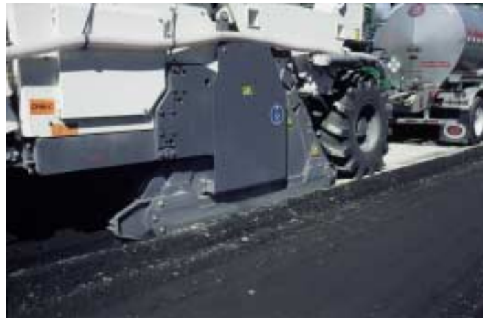
Portland cement is mixed in foam-stabilizing stages; operation moves from left to right
