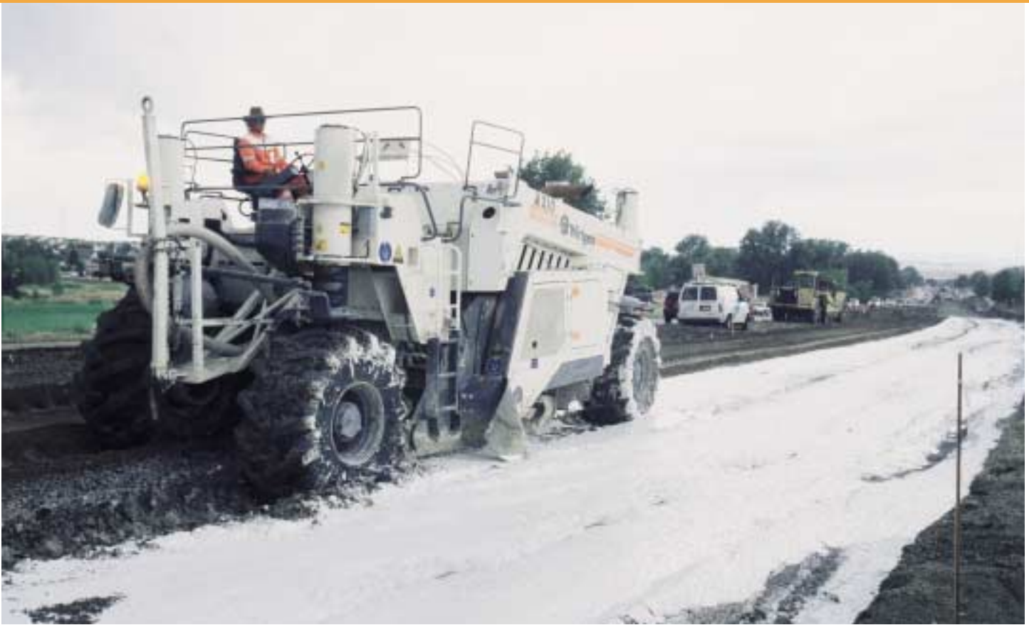
In Parker, Colorado, ARS lime-slurry stabilizes Main Street in reverse
