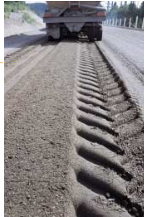
Base awaits compaction
