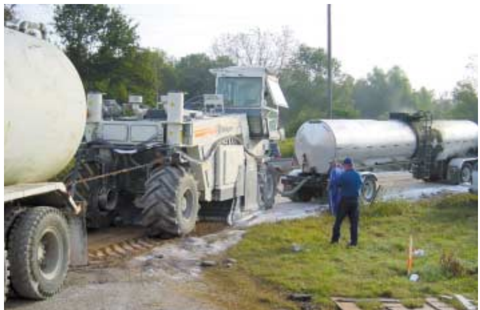
Foamed asphalt base recycling has potential to replace soil-cement bases in Louisiana
