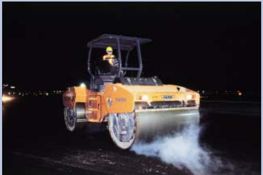
Paving would cease at 3 a.m. to permit runway to cool down
