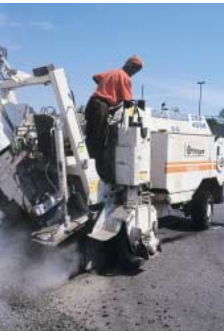
Wirtgen Model 1000 DC mills South Yosemite patch cuts
