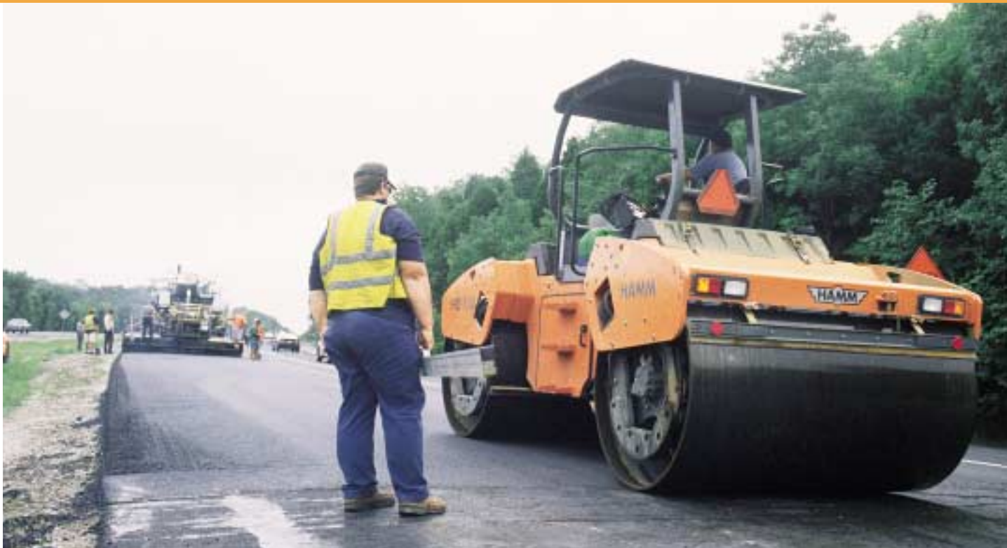
Hamm HD 130 provides initial compaction of mat
