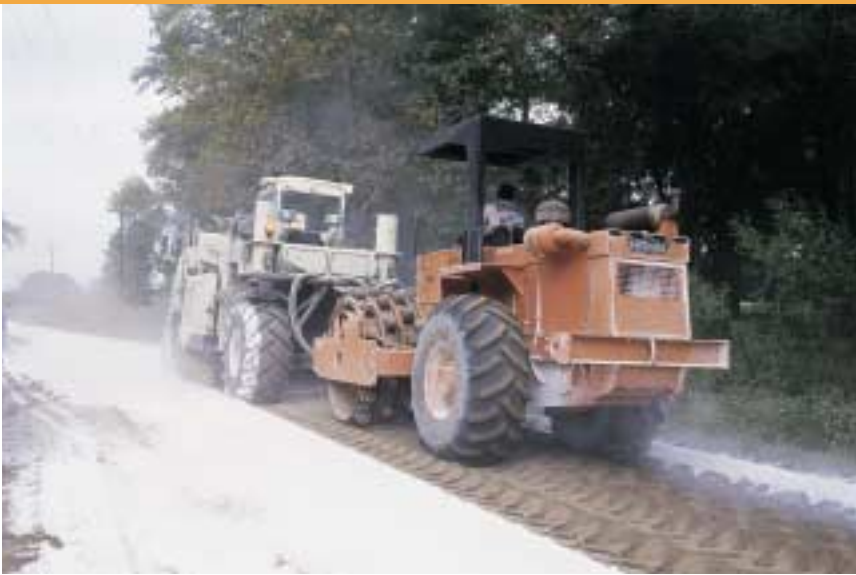
Hydrated lime was spread at 112 lb. per cubic foot of soil
