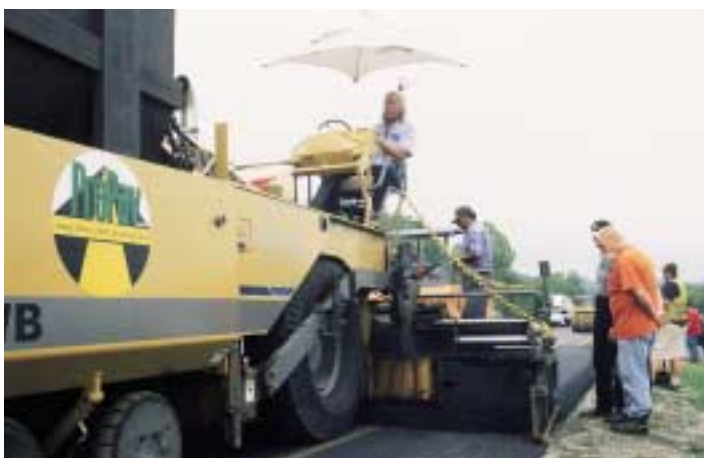
Pro Pav 1110 WB paver followed milling by W 2200 and W 1900 DC
