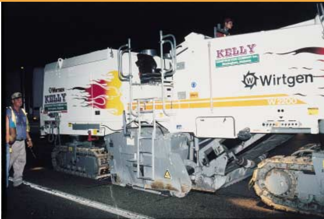
W 2200 is ideal for large-volume night work on I-65 in Alabama
