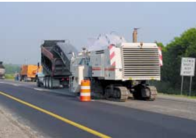
12.5 ft. cold milling preceded paving and compacting with Wirtgen Group products
