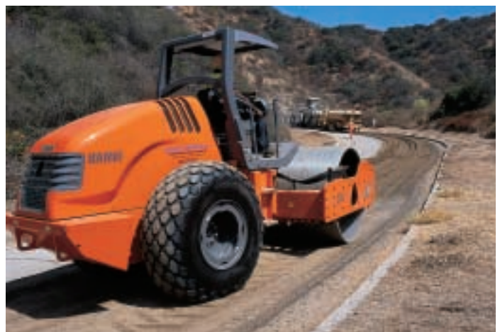
Hamm 3412 soil compactor follows recycling train up hairpin turns
