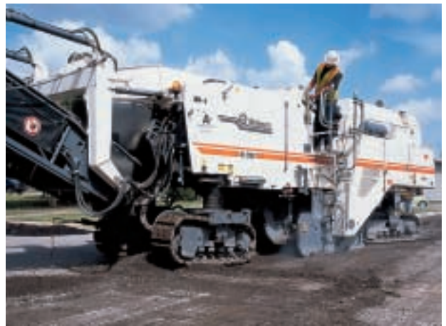
Separately steered 'legs' help W 2100 mill around concrete islands, enhance stability
