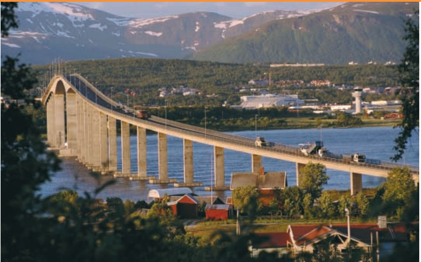
Nonaggressive oscillation compaction was used to place hot mix asphalt decks on major bridges in northern Norway; conventional vibration compaction not permitted on bridges by federal law
