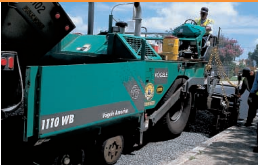
Eighty percent of work is maintenance, including mill and overlay
