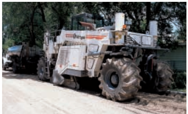
San Antonio's WR 2500 reclaims residential street
