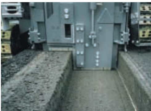
FCS with drum width of 24 inches at work on W 1200 F
