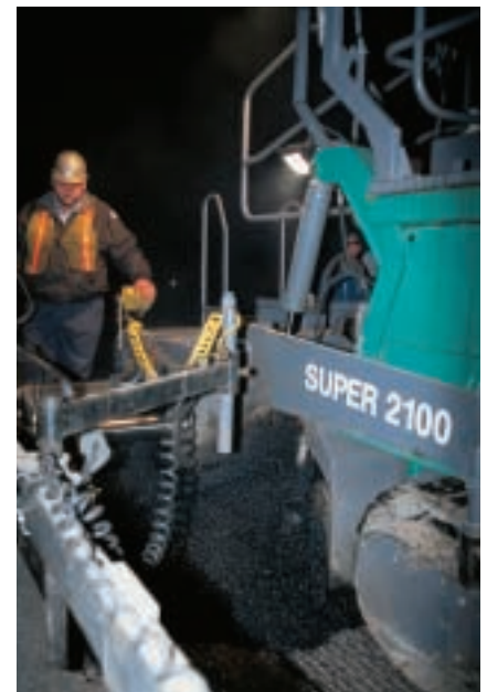
Vögele Super 2100 places SMA on U.S. 17 near Fredericksburg, Va.; compaction at screed is in the high 80s
