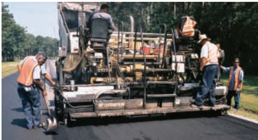
Older MAC 1110 T places Superpave on private community golf course roadway north of Myrtle Beach
